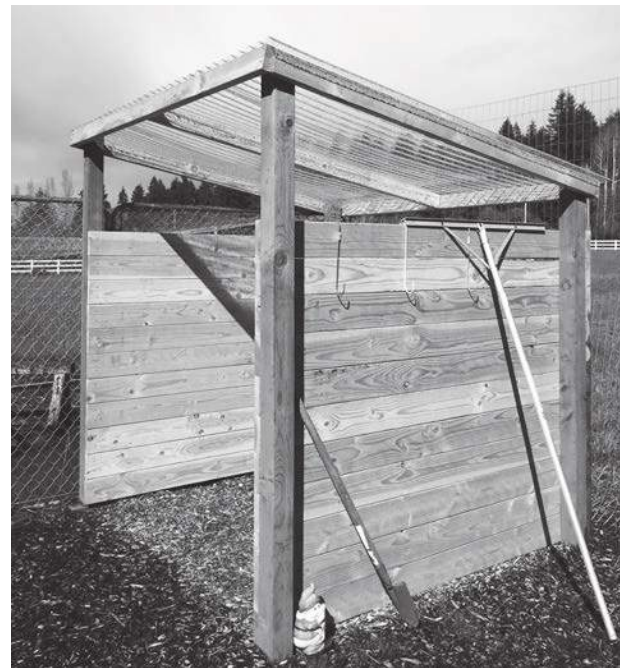
Livestock owners can build a manure bin for less than $500 in materials. Courtesy Pierce Conservation District
