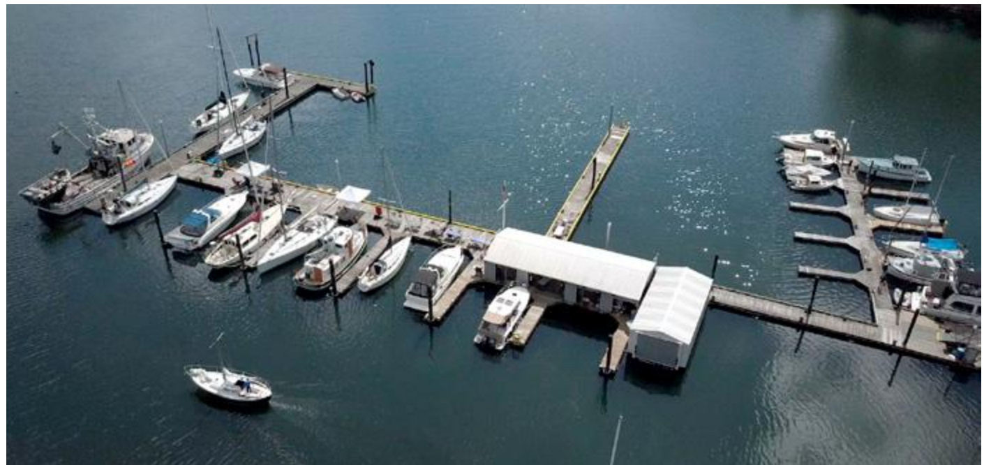
The popular Filucy Bay facility will use state funds for long-needed repairs and improvements.. Photo courtesy Kelly Guenther
