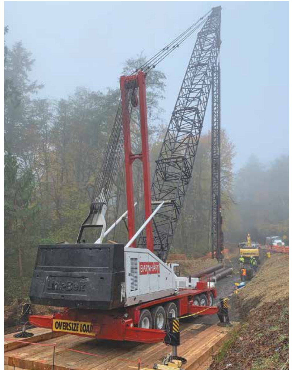
Bridge bypass under construction in November. Photo: WSDOT
