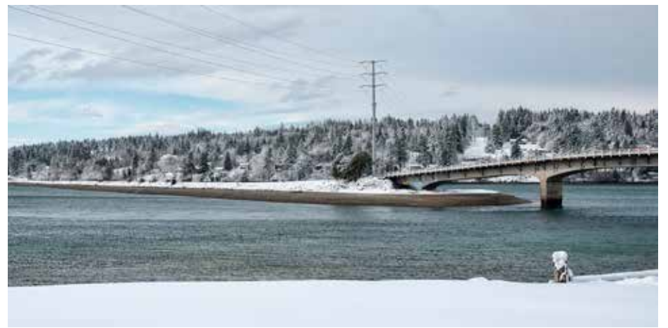
The year started off with a bang when the Puget Sound region saw 20.2 inches of snowfall in the first half of February, the most in 50 years. It made for scenic views and long hours for Peninsula Light Co. crews struggling to keep up with powerlines downed by falling trees. "Snowmageddon" left a lasting impression, as Pen Light spent most of the summer trimming trees and replacing lines along the Key Peninsula Highway and State Route 302. Top photo: Beth Buffington, Above: Ed Johnson, KP News
