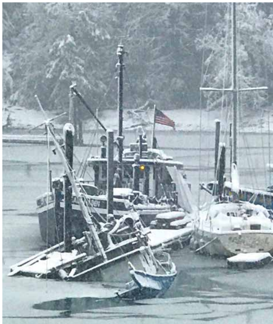
Heavy snowfall and tidal action combined to shift the sunken boat under its dock, threatening the marina structure. Photo: Lisa Bryan, KP News
